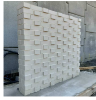
4. PROTRUDING BRICK DETAIL
