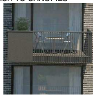
10. CANTILEVERED BALCONY WITH PPC VERTICAL RAILING
